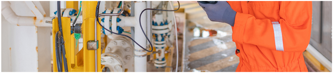
FIG. 1. Traditional instrument configuration and troubleshooting tasks must often be done at the device, raising safety and other concerns due to extensive time spent in hazardous, and often difficult to access, areas.
