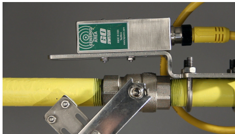
Figure 22: Safety Shower Valve in Activated Position
